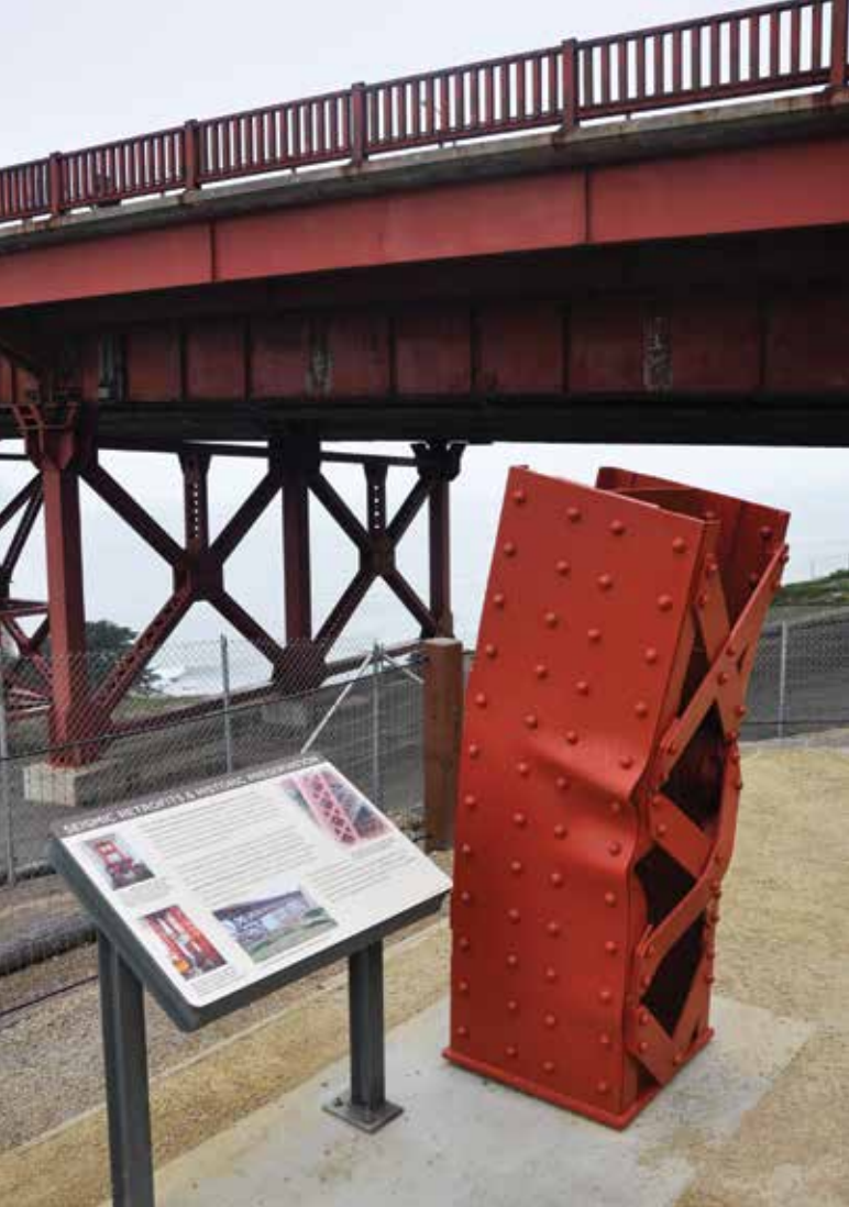
This portion of a tall strut was made identically to one of the original struts on the bridge and then tested in a University of California civil engineering laboratory. Photo courtesy Golden Gate Bridge, Highway and Transportation District
